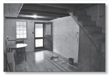
D8 and D9 received a few repairs and a fresh coat of paint also. The interiors of these cabins are receiving a much needed face lift in the form of updated wiring and updated furnishings when needed. The walls are being finished with insulation and an application of pine wood
